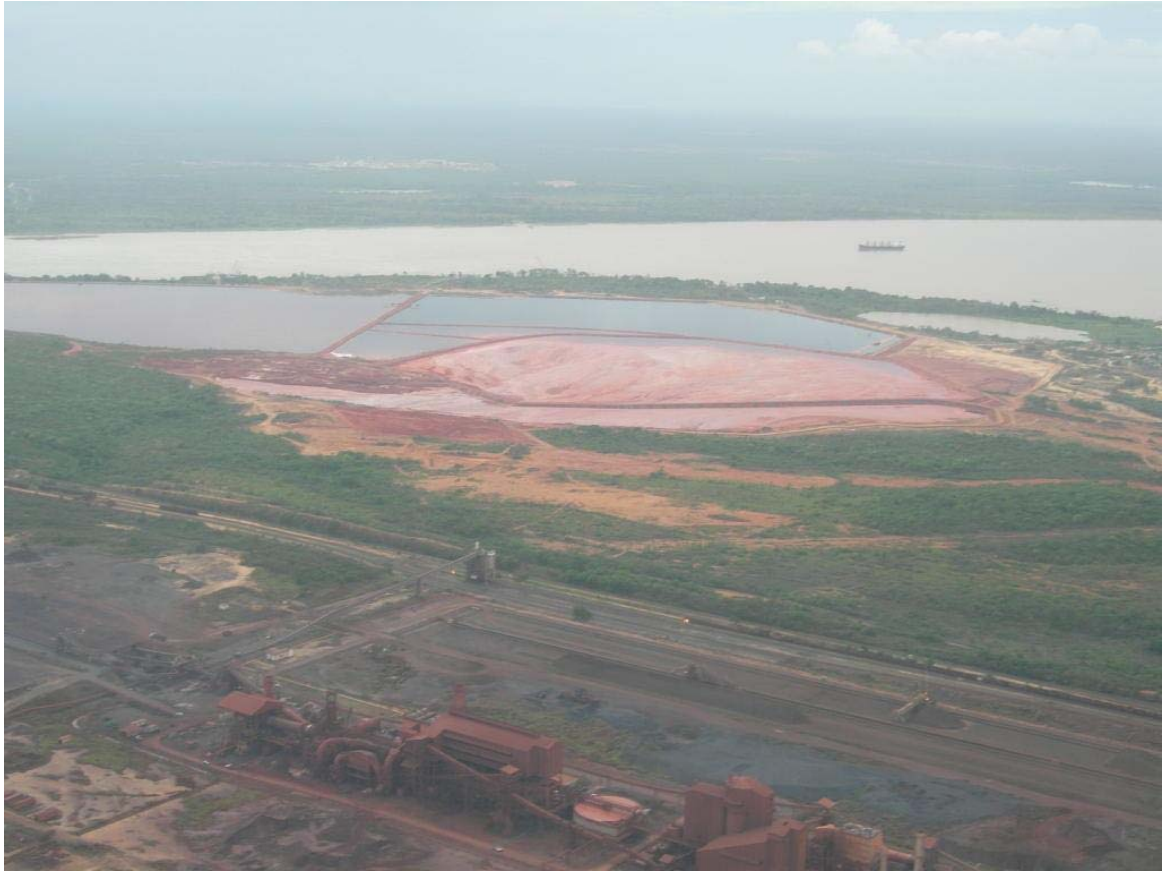
Figure 7 - Iron Ore Plant for Ferrominera and tailings impoundment at Puerto Ordaz, Venezuela on the edge of the Orinoco river. Looking North. Photo SDO, 1 June 2005.
